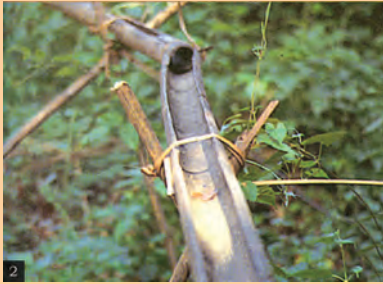
Picture 2 and 3: The channel sections, made of bamboo, divert water to the plant site where it is distributed into branches, again made and laid out with different forms of bamboo pipes. The flow of water into the pipes is controlled by manipulating the pipe positions.
