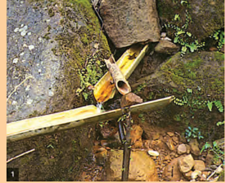
Picture 1: Bamboo pipes are used to divert perennial springs on the hilltops to the lower reaches by gravity.
