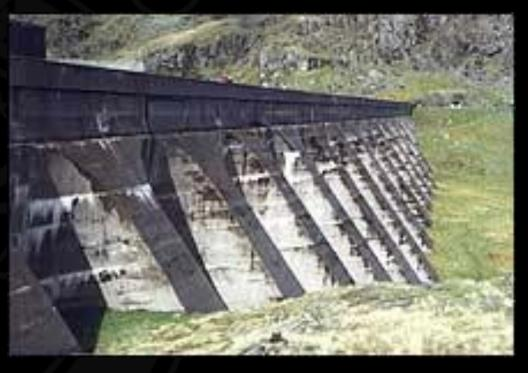
The buttress dam was developed from the idea of the gravity dam, except that it uses a lot less material due to the clear spaces between the buttresses. Like gravity dams, they are suited to both narrow and wide valleys, and they must be constructed on sound rock.
